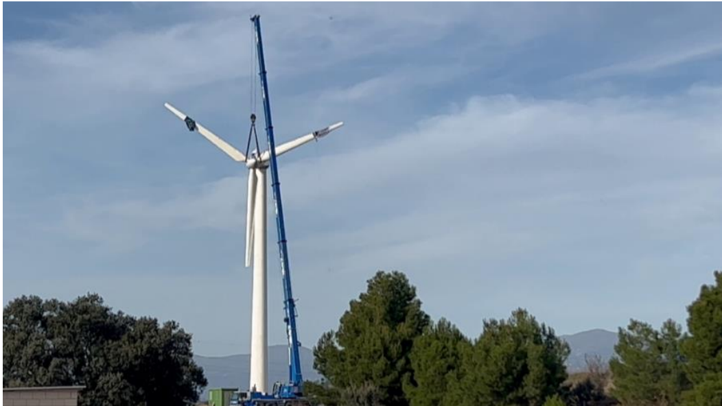
Figure 5. Wind turbines installation (2024)
